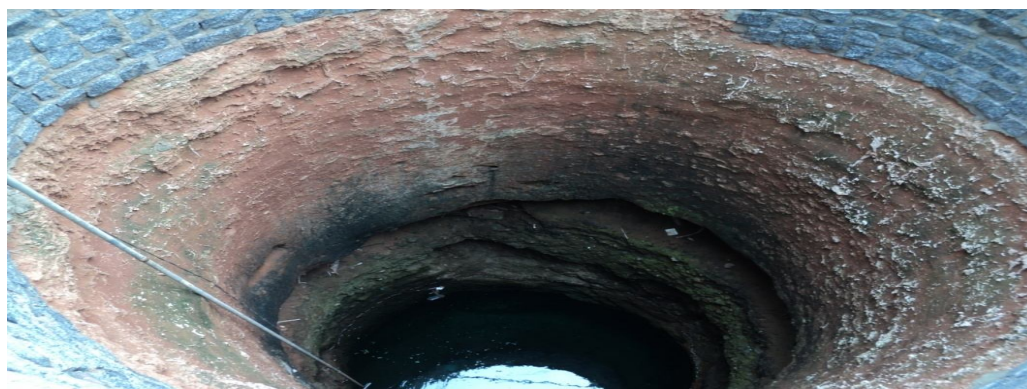
Fig.11: Depth of weathering in the observed well at Periyankuppam village (Long 78.670 Lat 12.752)
