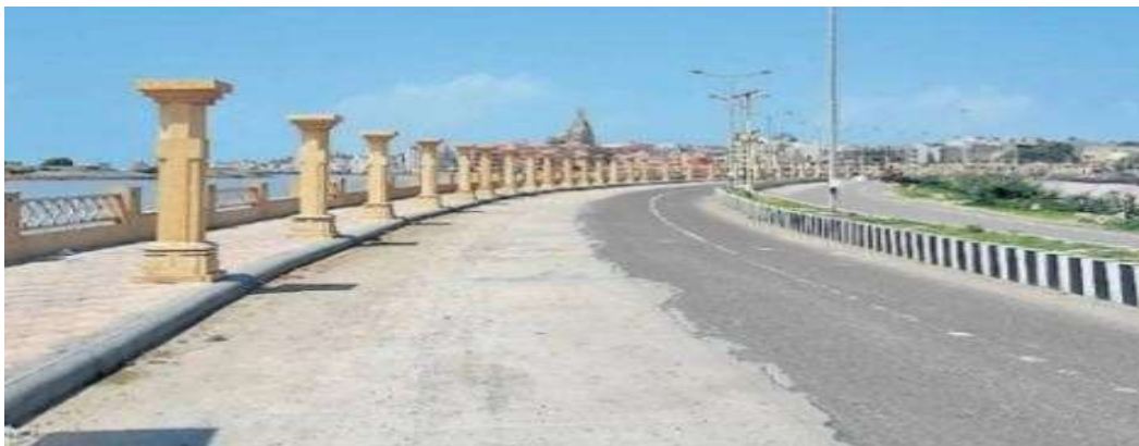
Figure 5: Works done in Dwarka city a) heritage structures and Seaside development. Source: Author
