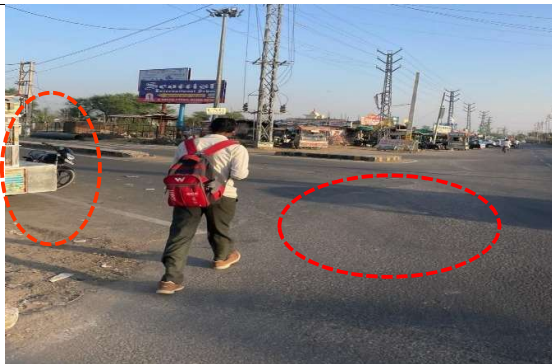
Fig. 5 Shows the Blackspot Location Rajgarh Road Naka which shows that there is no pedestrian crossing marking and no signal light for this T-junction. There is no Give Way sign board and no junction marking. The sight distance is not clear at the corner of the conflict point.
