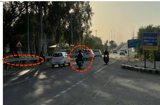
Fig. 4 Shows the Blackspot Location South Bypass Sector 16/17 which shows that there is no median between two lanes of road, vehicles are overtaking in opposite lanes, restricted overtaking zones are not available, and reflecting lights or paint on side brigades are not available.
