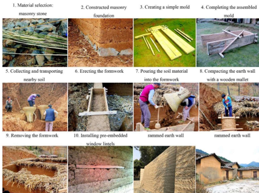
Figure 4: Construction process of rammed earth walls: site selection and material preparation; building the foundation,
