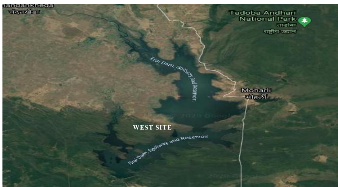
Fig. 1. Satellite View of Erai Dam, Chandrapur Maharashtra, India
